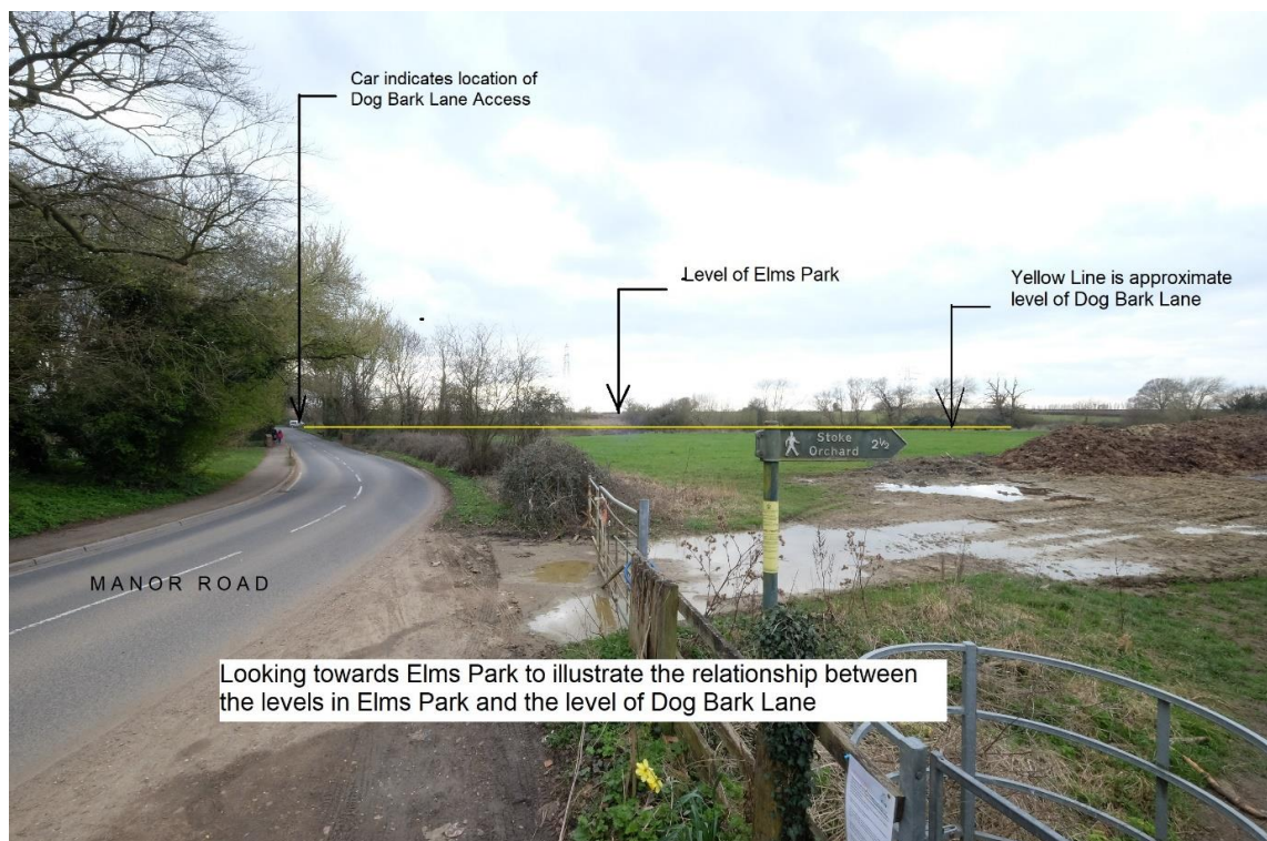
Figure 1: View south from Manor Road towards Dog Bark Lane and Elms Park.
